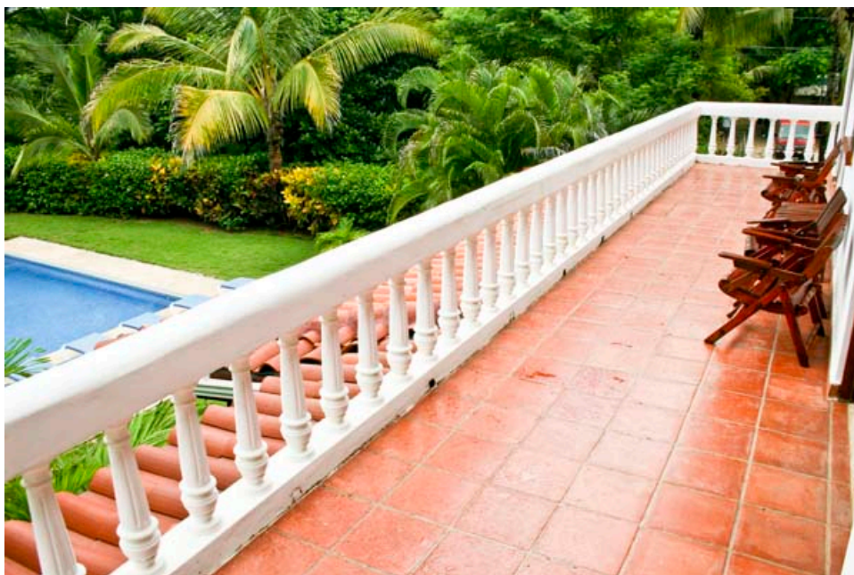
Oceanside Balcony Outside the Master Bedroom and Bedroom 3
